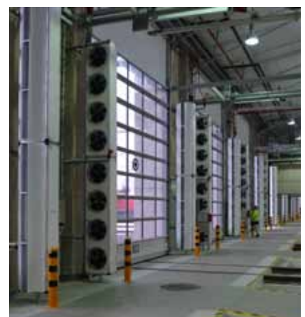
Max Multiple towers on large industrial doors
